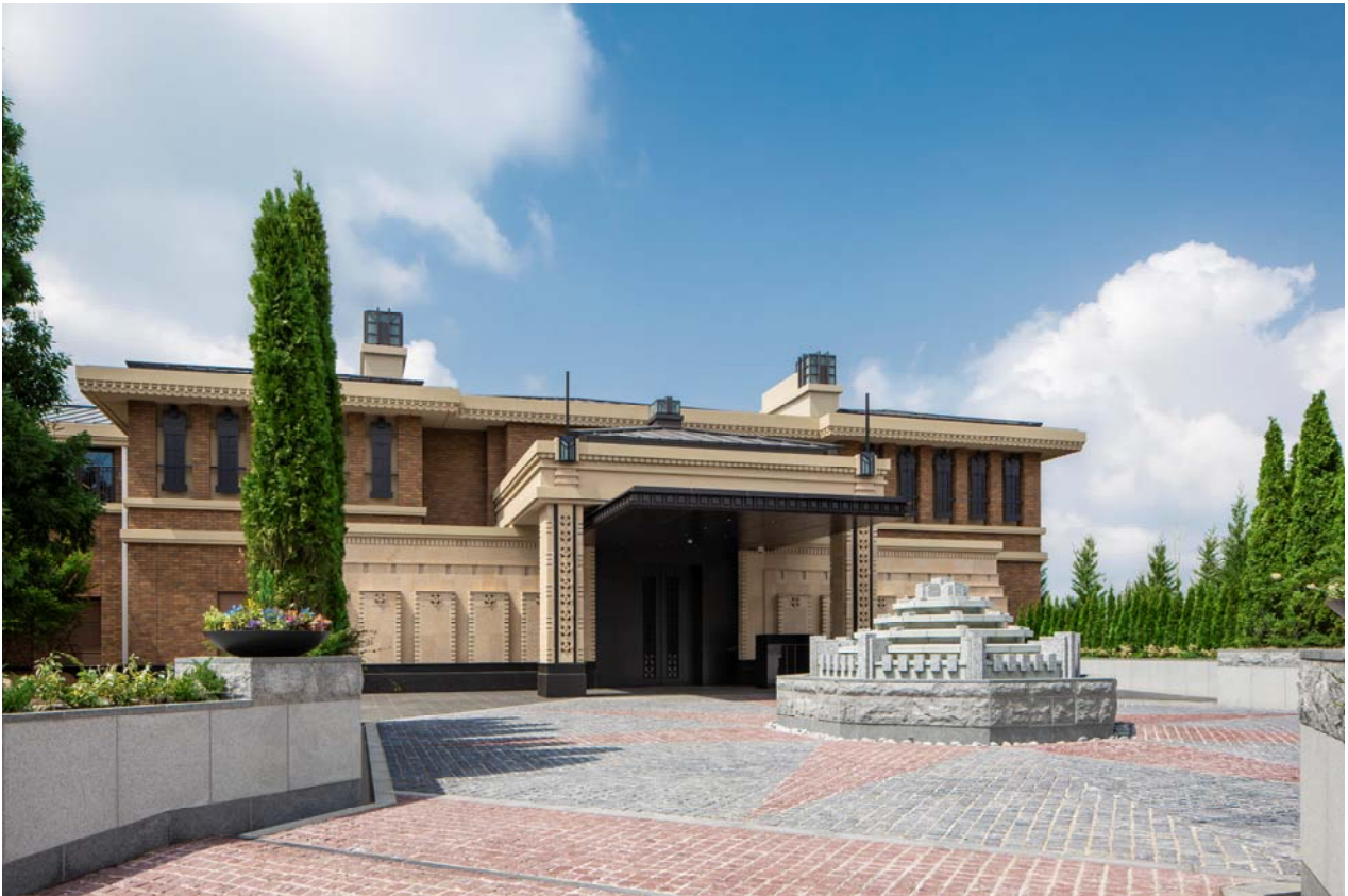
View of the “Center Building” from the “Portecochere”
