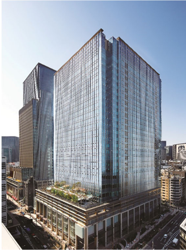
Nihonbashi Muromachi Mitsui Tower Exterior
