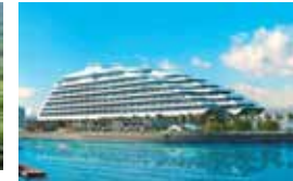
Opening in February 2018 Ashiya Baycourt Club (201 rooms)
